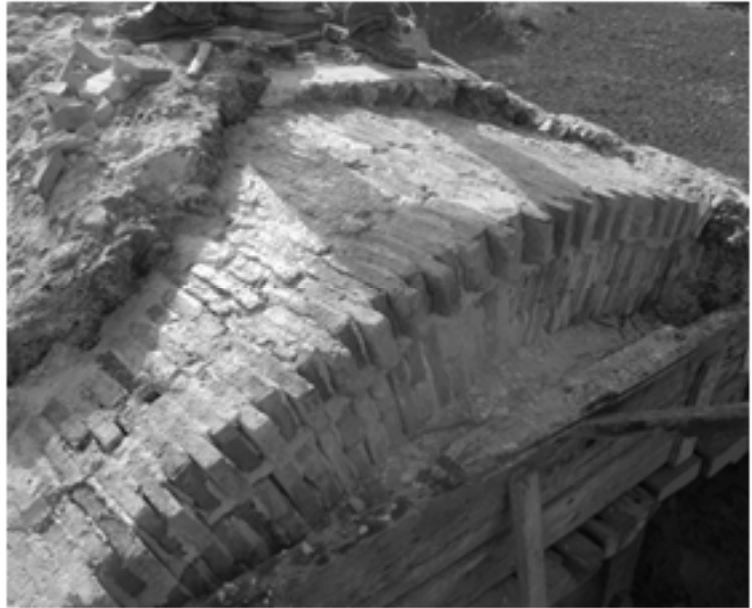
Fig. 8 The bricks used in the reconstruction (A el H)
