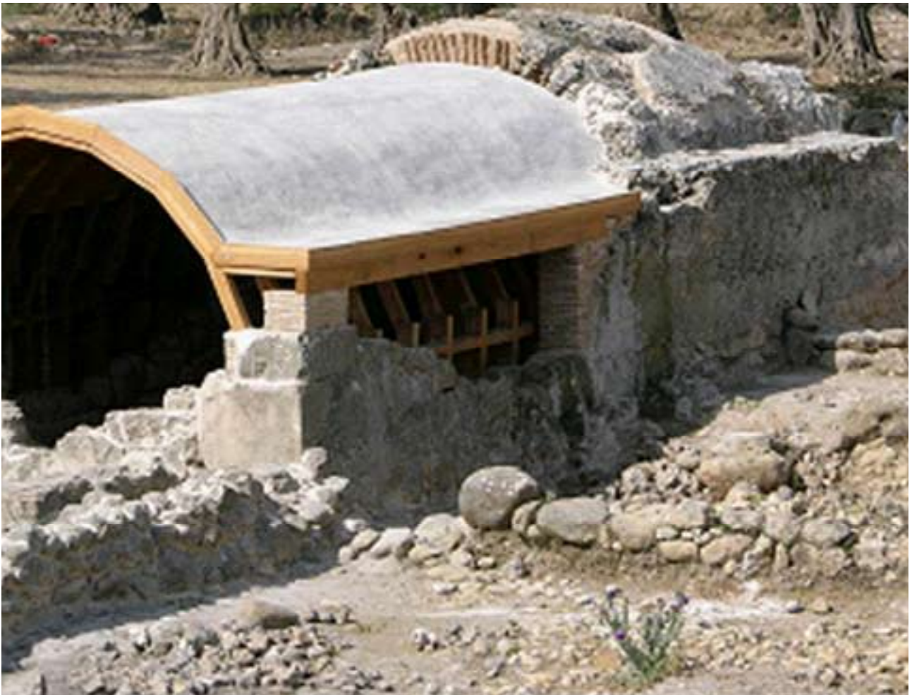
Fig. 11 The wooden vault covered with planking and waterproof membrane (A el H)
