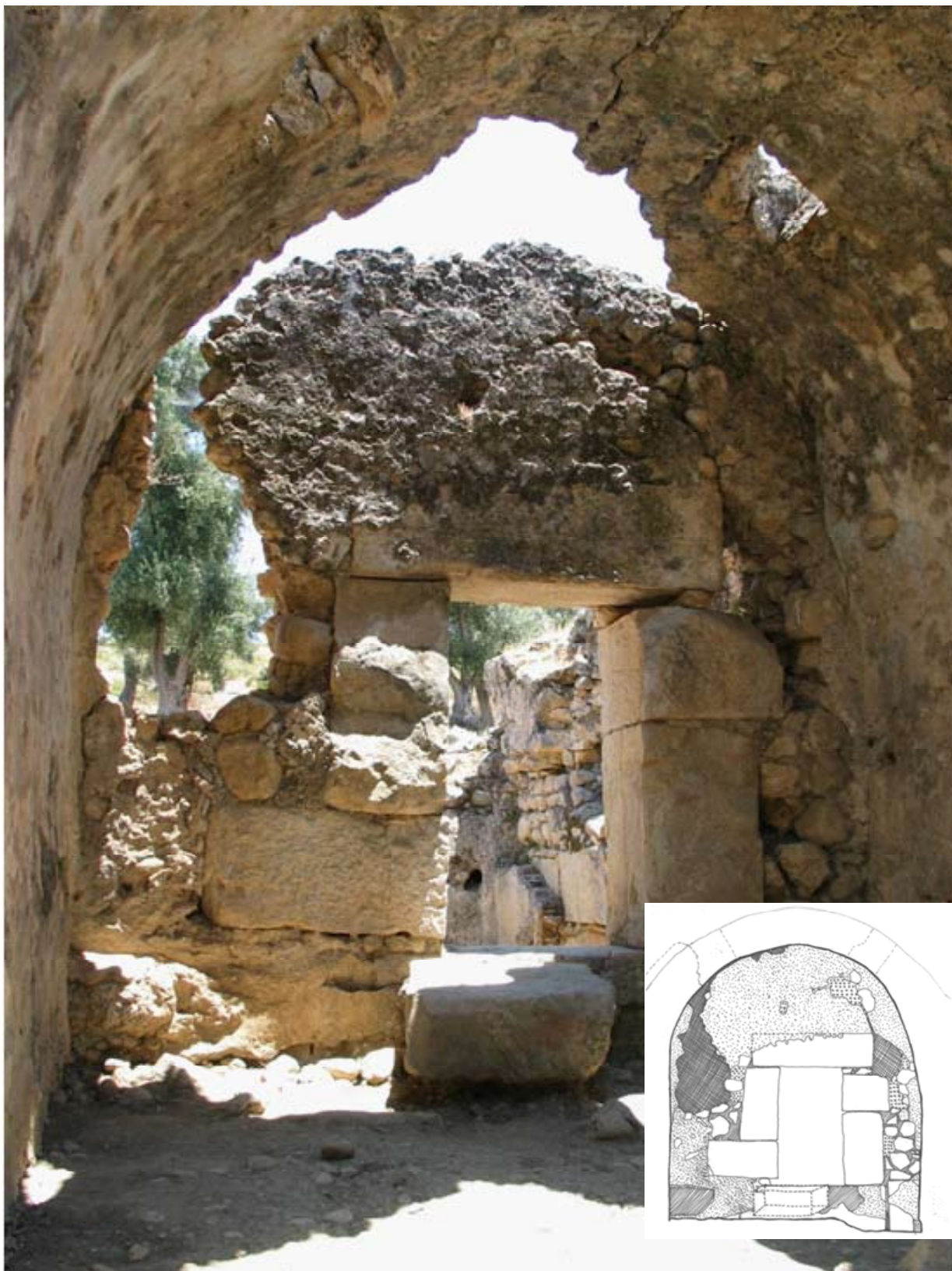
Fig. 5. Room IV, from the east and Fig. 6. Documentation of Room IV (A.el H)
