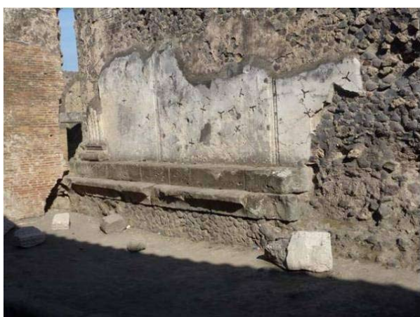
Fig.12. Clamps securing the plasters in the rear of the Capitolium.
