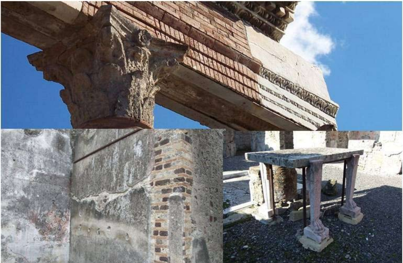
Fig. 24. The use of iron in restorations: chains, lintels, supports.
