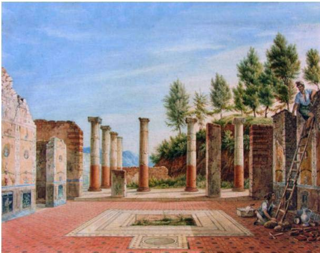
Fig. 10. Workers putting a tiles cover on the top of the walls (L. von Zanth, ca 1822-24).
