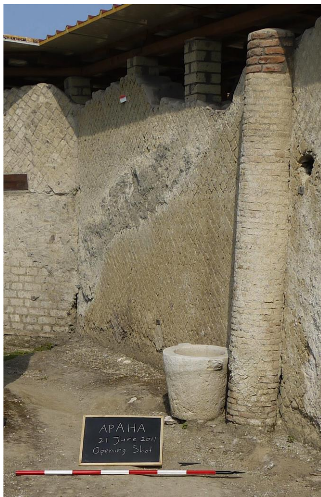
Fig. 7. Room 68, northwestern corner. Limestone mortar.
