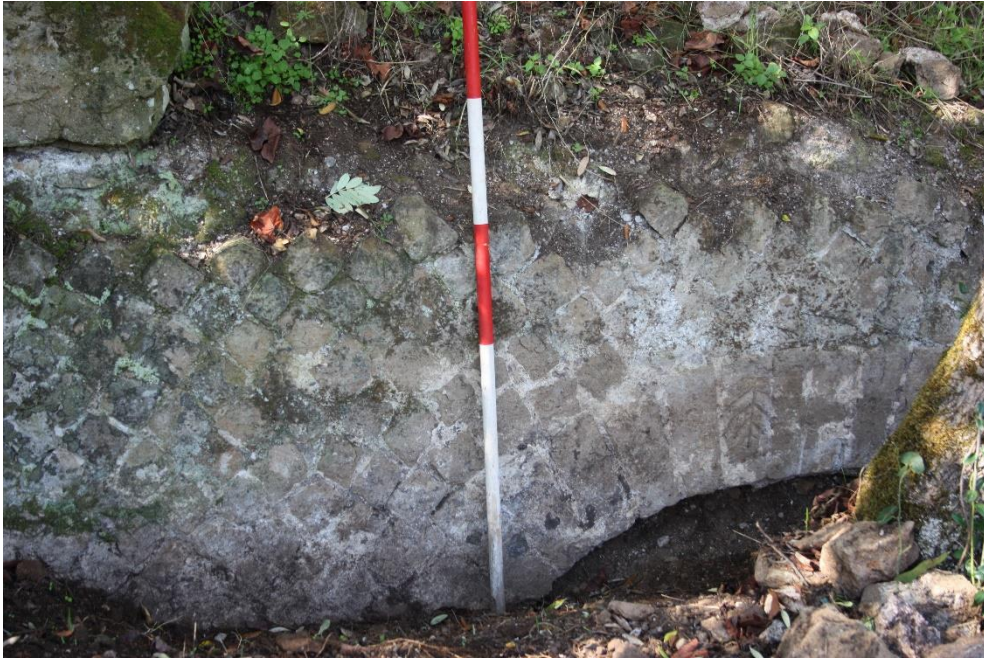
Fig. 7. Cleaned arch of aqueduct north of cistern in proprietà Colleoni, with palmette incised on key-stone (2012).
