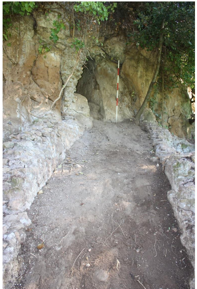
Fig. 11. Opening in the hill-side of late Republican aqueduct and below walls for outlet of water, viewed from the west.
