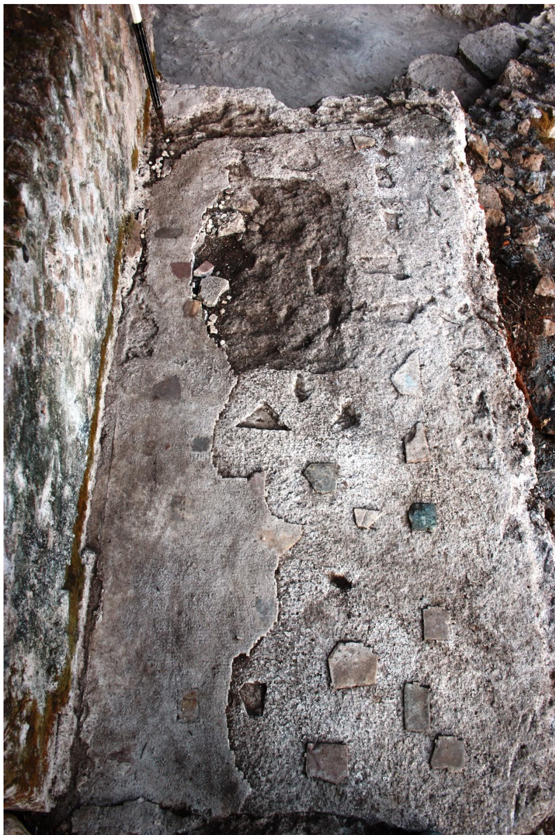
Fig. 14. Building A, mosaic floor with crustae of marble to the west of the basin. Probably late Republican.
