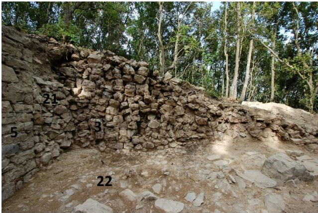
Fig. 8. Area 1000: the western façade of the curtain wall 3. Also visible in the picture the walled-up door 21.
