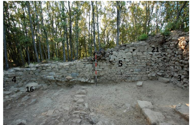
Fig. 9. Area 1000: southern façade of wall 5, with the walled-up door 21.
