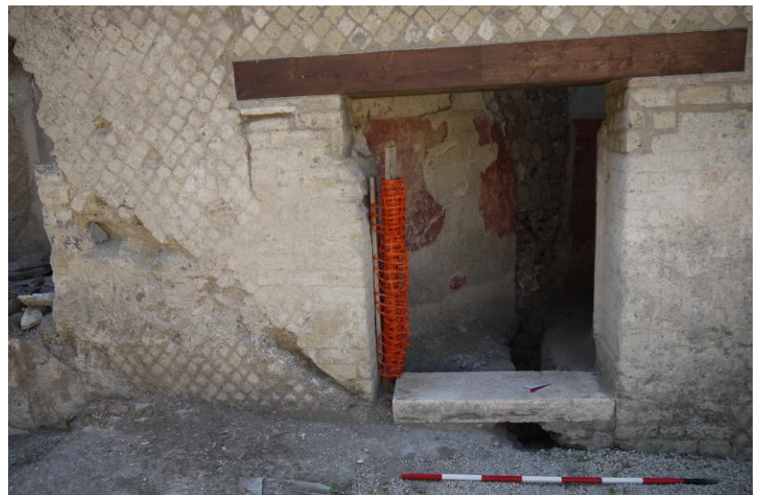
Fig. 4. Entrance to southern latrine, with Bourbon robber cut visible underneath threshold, leading to cuniculus (repaired in modern times) in wall in the back, separating latrine from 'palaestra'.
