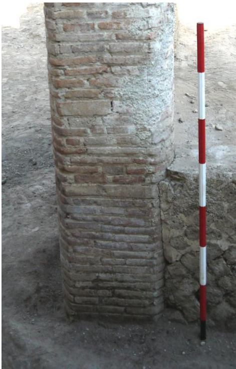
Fig. 15. Northwestern pier of colonnaded open space looking east, showing rounded sides on north and south, flat side towards west.
