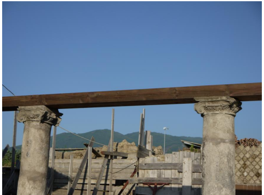
Fig. 16. Trench 1000. Extended colonnade, looking east. Carved capitals in gray tufa on top of columns.
