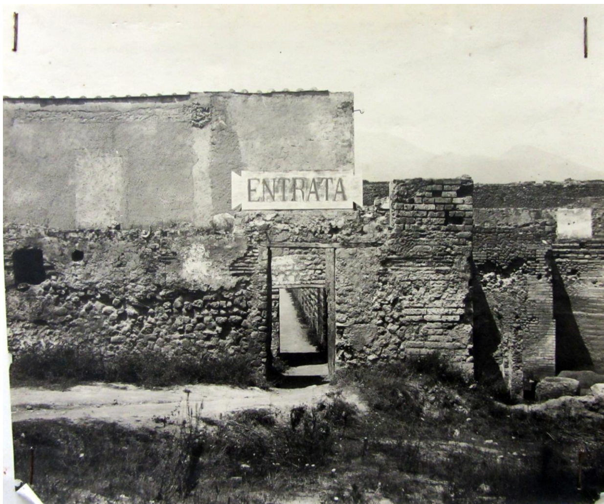
Fig. 1. Former entrance to the Quadriporticus . (Soprintendenza Antichita Napoli, #7950). Undated, but likely 1941.
