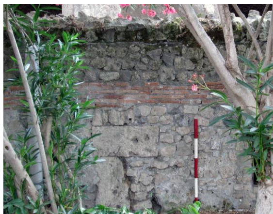
Fig. 8. Phase one Sarno limestone construction in WF 219.
