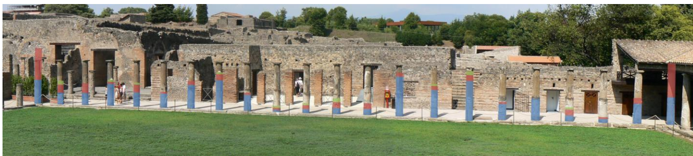
Fig. 4. Column graph of interventions on columns of eastern portico.
