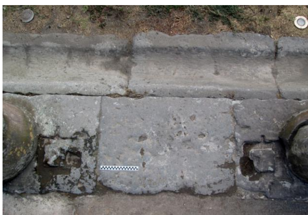
Fig. 5. Cuttings at the center intercolumniation of east portico.
