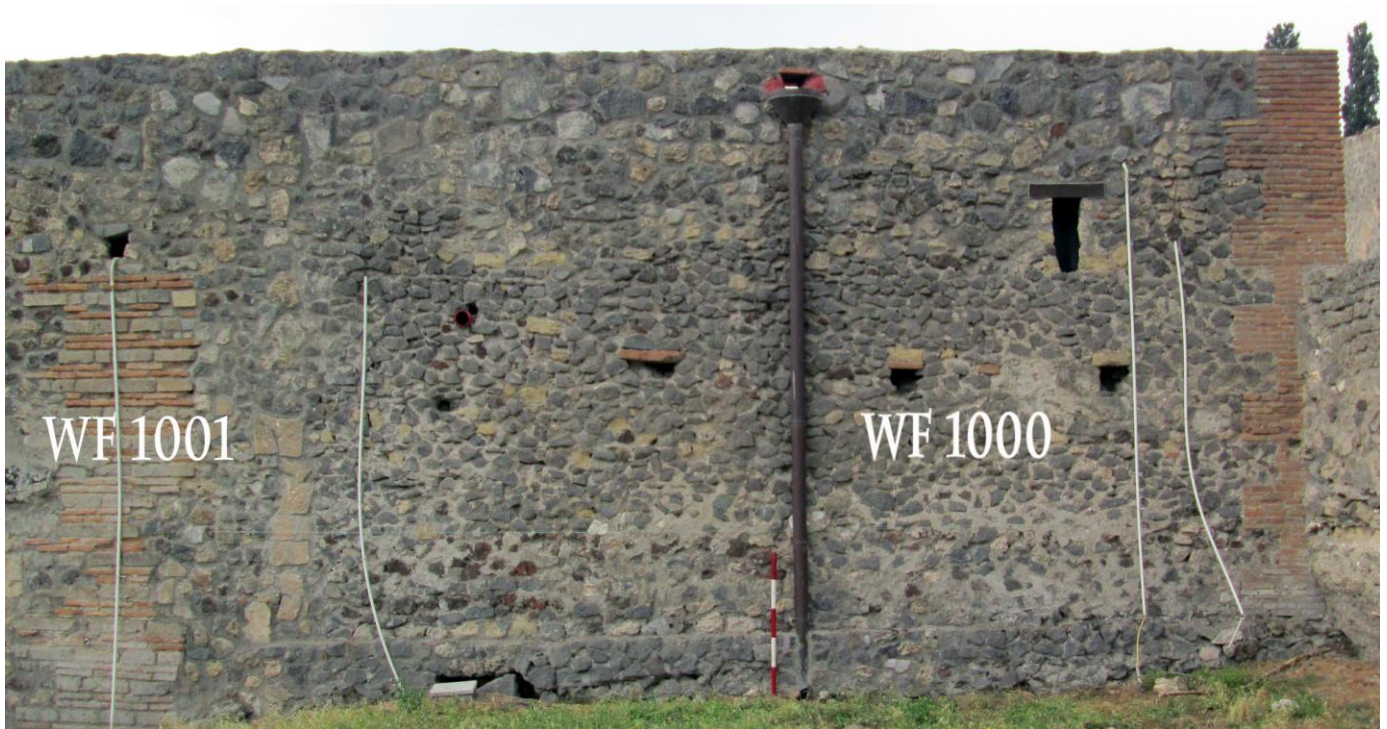
Fig. 12. Phase three opus incertum construction in WF 1000.
