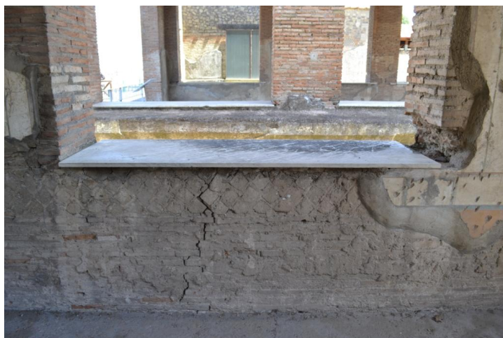
Fig. 19. Villa Arianna , Room 3, modern windowsill replacement. The restored sill is shorter than the original marble.
