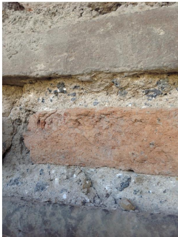
Fig. 9. Mortar Detail, Wall Face 172, SU 172.003.
