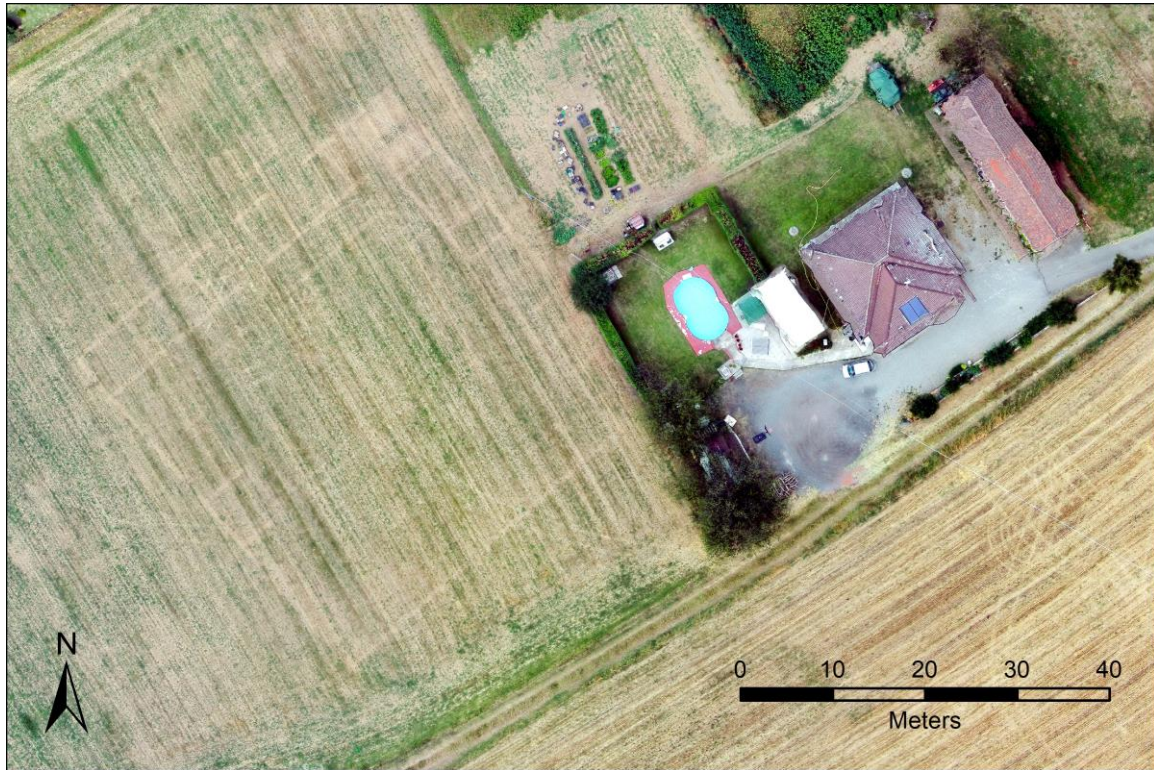
Fig. 7. Satellite image of large building in Field Q. Map image: Google Earth.
