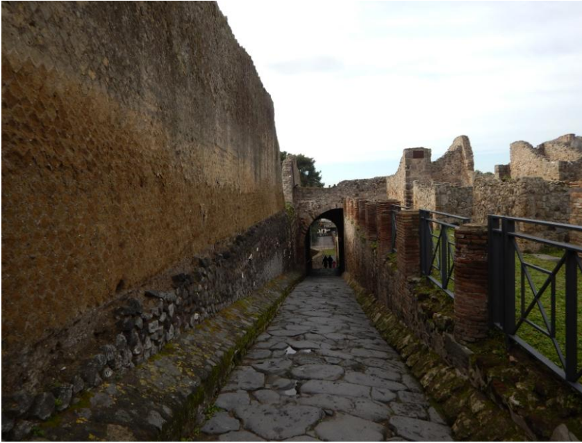
Fig. 18. PPT 2015-16 project, view of via Marina from E. To the left is visible the Yellow Neapolitan tuff opus reticulatum precinct wall of the Sanctuary of Venus (10) on top of the pre-existing lava opus incertum terracing structure (18).
