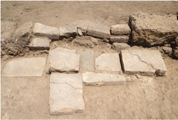
Fig. 25. Doorway between Walls H and H1 leading from Plateia B into Room 2a, looking north.
