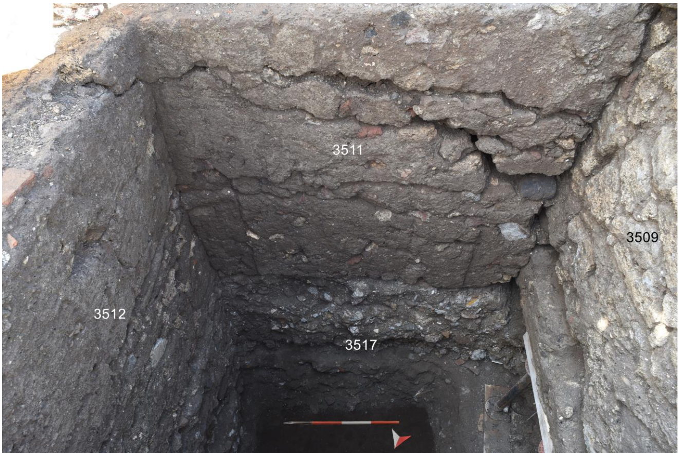
Fig. 22. VPP 2019, Trench IVN, concrete substructures of the cella. Detail of the E-W wall 3511. Note how the wall is built in two courses, with the lower section preserving traces of the formwork. The structure rests directly on top of the construction fill 3517 (the upper portion of which was excavated by Curti) (Photo: VPP). To the left is visible the N-S grid wall 3512, featuring a similar technique; to the right is the podium retaining wall 3509 (the upper portion of which was raised without shuttering).
