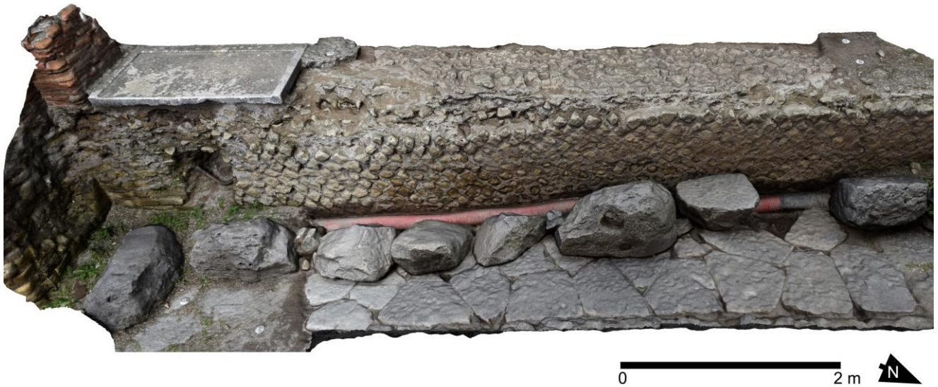
Fig. 26. VPP 2019, Trench C: Composite photomodel of the Flavian-era precinct wall (12008), viewed from E. Note the marble sill, at much higher elevation than the pavement of the N-S leg of the Vicolo di Championnet, and the spoliated basalt pavers (Author: D. Diffendale).
